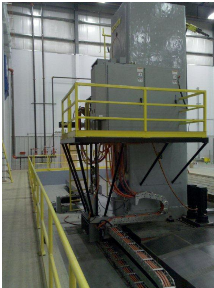
Main enclosure install on back of machine.
